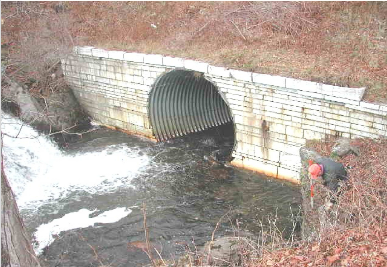
Upstream end – Existing Marble Masonry Headwall
